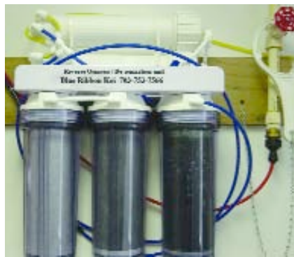
A small RO unit can deliver about 200 gallons of perfect water every day!
