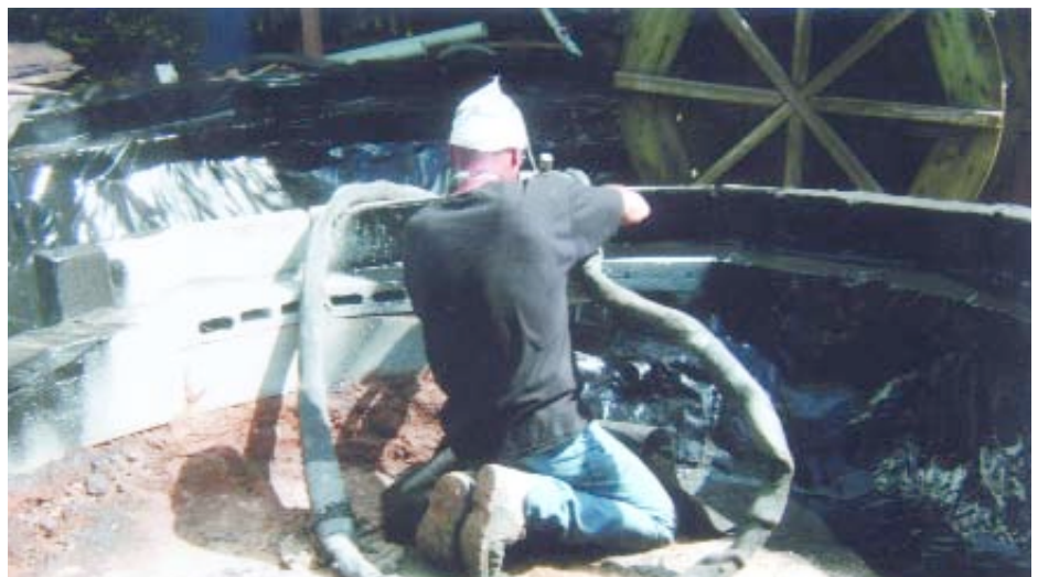
Kerry spraying the liner.
