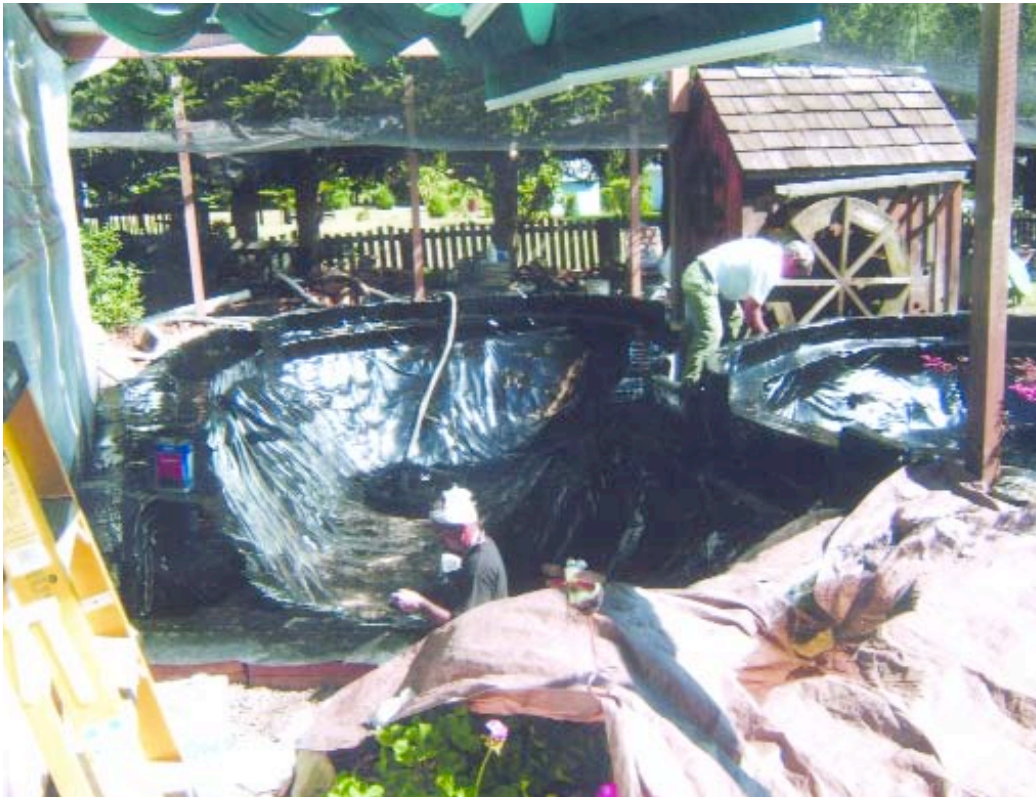
Kerry and Terry checking their work.
